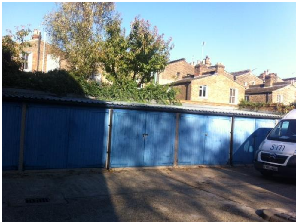
Photo 5: Rear garages to be demolished
