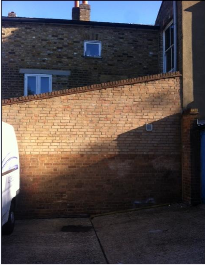
Photo 6: Neighbouring property No.138 Thorpedale Road
